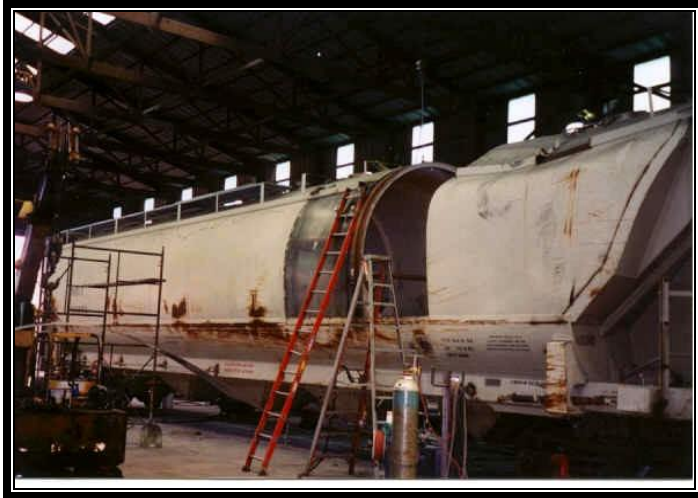
Reconstruction of a Covered Hopper Railcar BEFORE
